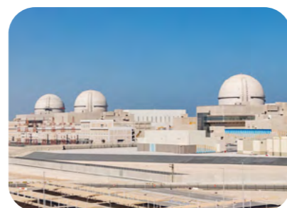
Hanmaek Power Plant - South Korea
