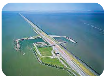
Excavation in IJsselmeer - Netherlands
