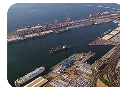
Service Harbour - Fujairah, UAE
